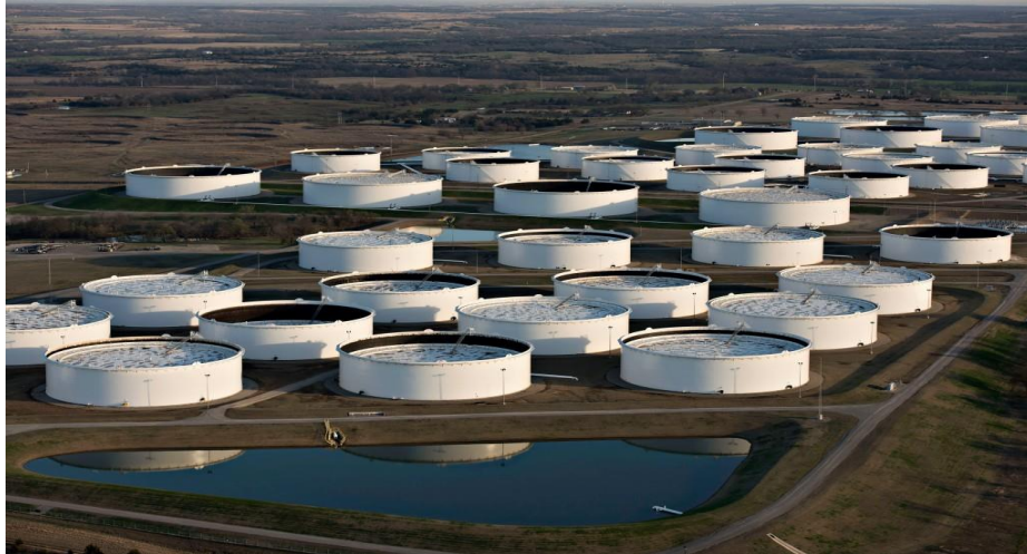
Picture 12. Tank farm
