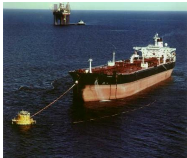
Picture 15. Single buoy mooring
