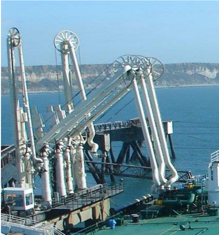
Picture 16. Marine loading arm
