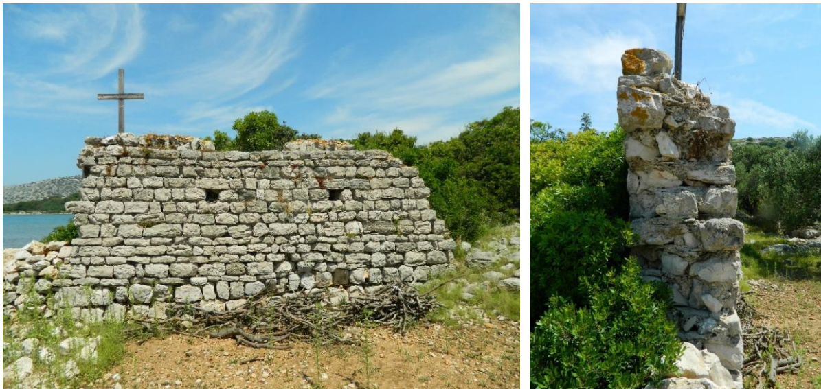
Fig. 196 Medieval wall that possibly belonged to a salt warehouse (M. Grisonic).
