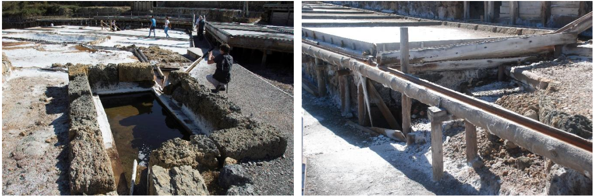
Fig. 5 Salinas de Añana: brine storage well and brine channels (courtesy of Alberto Plata and Noelia Tofé).
