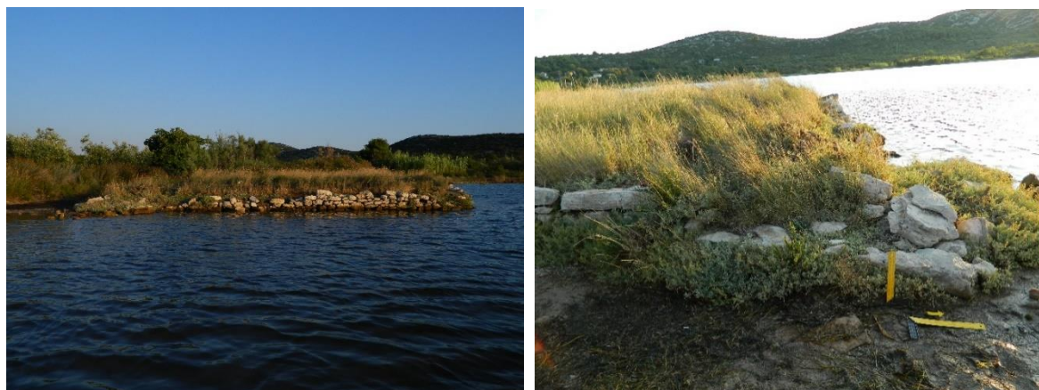
Fig. 136 Big dry wall structure on the coast – a salt warehouse?: the N side (a) and its NE corner (b) (M. Grisonic).
