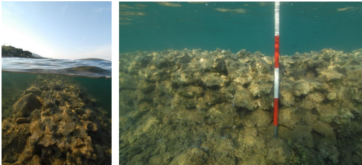
Fig. 167 Western separation wall (Wall 3) (M. Grisonic).
