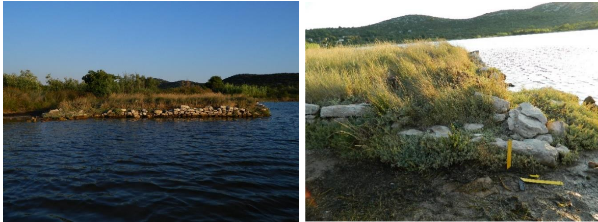
Fig. 136 Big dry wall structure on the coast – a salt warehouse?: the N side (a) and its NE corner (b) (M. Grisonic).
