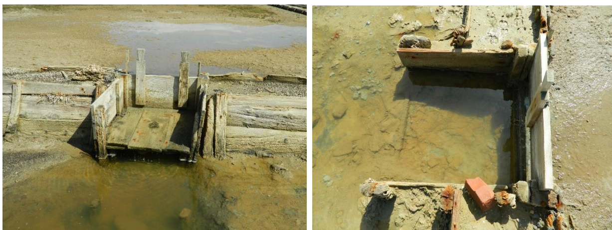
Fig. 58 Sluice gates in between the salt evaporation pools on the saltpans of Pag (M. Grisonic).
