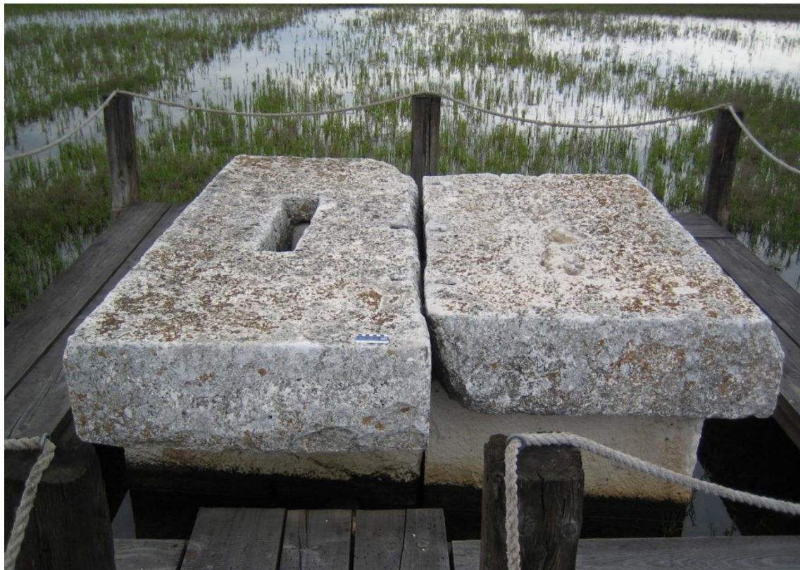
Fig. 69 The so-called Roman sluice gate on the salt pans of Nin (M. Grisonic).
