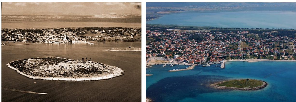
Fig. 209 a: Mid-20th century aerial picture of Pakoštane with the still-existing Jaz Cove on the left side of the picture (Radić Rossi et al. 2018, p. 244).
