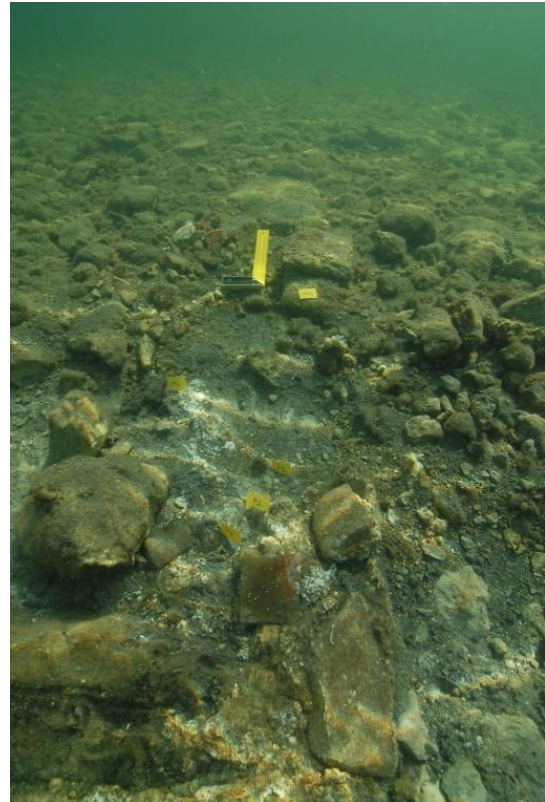
Fig. 123 Wall 6: in the foreground it is preserved at the level of foundations, while in the background a row of blocks still stands (M. Grisonic).
