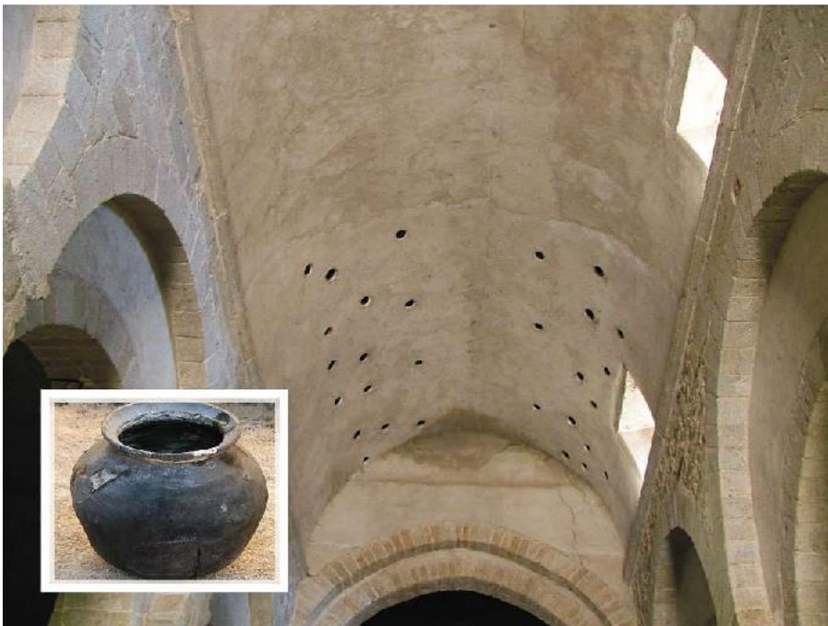
Slika 10. Akustične glinene posude u svodu crkve Pommiers en Forez, Auvergne (izvor: https://www.researchgate.net/figure/View-of-the-vault-in-the-nave-of-the-church-of-Pommiers-en-Forez-in-Auvergne-France_fig4_262853383 )
