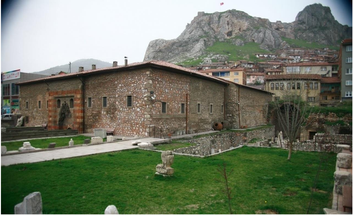
Figure 30 General view from the east
