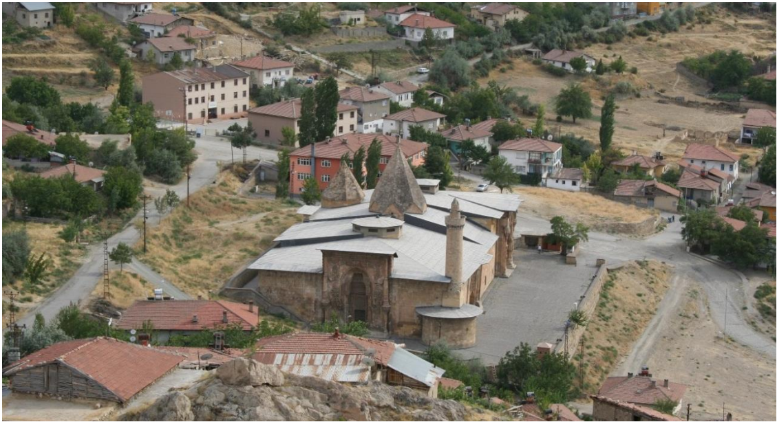
Figure 14 General view from the north
