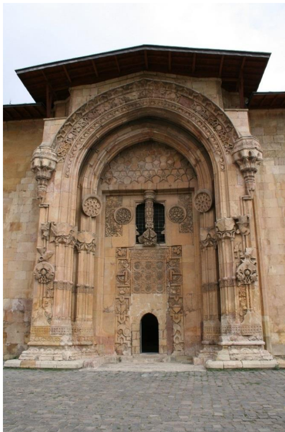
Figure 15 The main door of the hospital
