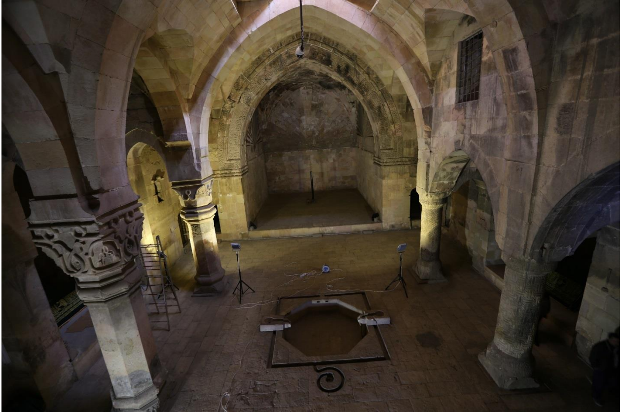
Figure 16 The main iwan and the pool, view from the west
