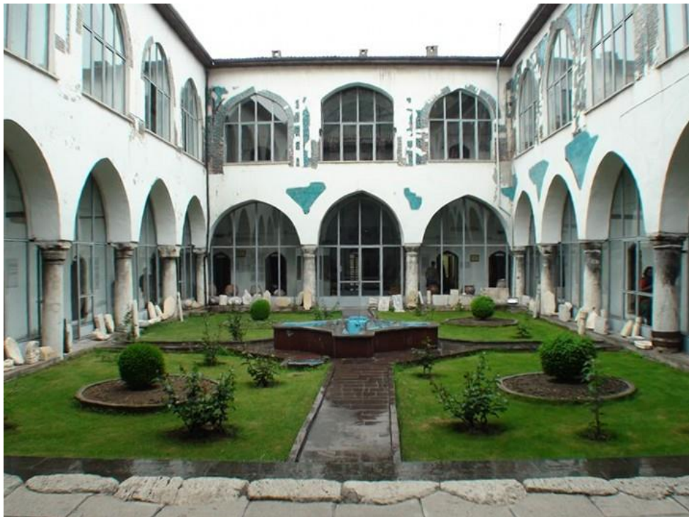
Figure 33 Open courtyard, looking at the east side
