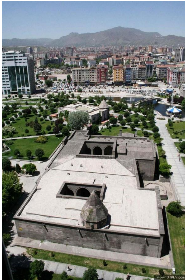
Figure 5 A general view from the east (Photo by Burhanettin Akbaş)
