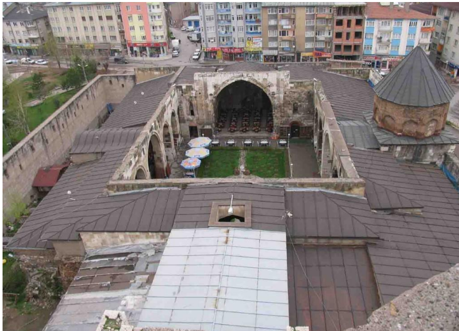
Figure 9 General view from the west
