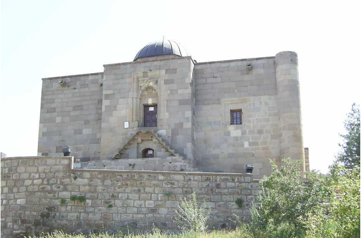
Figure 23 General view from the north
