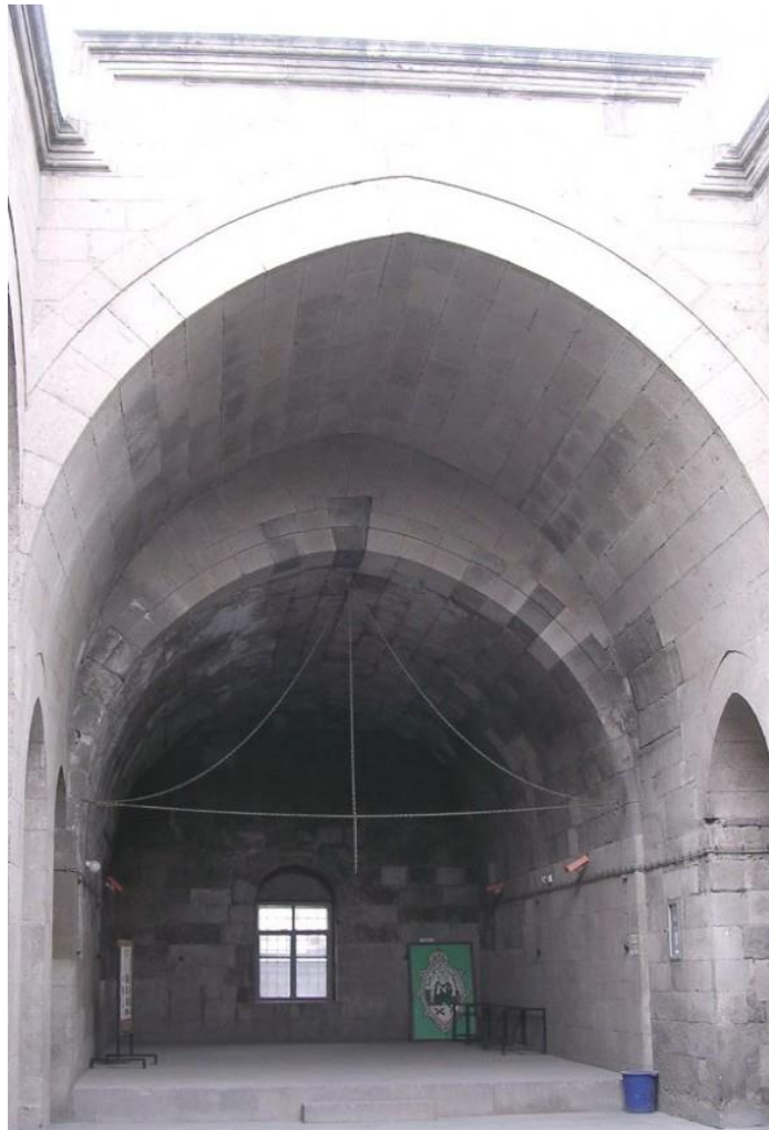
Figure 7 The main iwan, general view from the south
