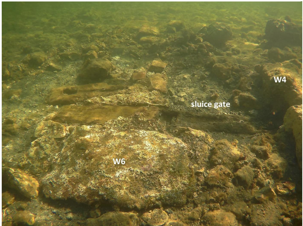
Fig. 113 Probable Wall 6 foundations and a sluice gate in between W6 and W4 (M. Grisonic).
