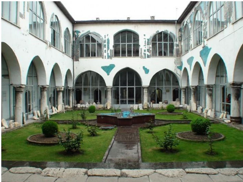
Figure 33 Open courtyard, looking at the east side
