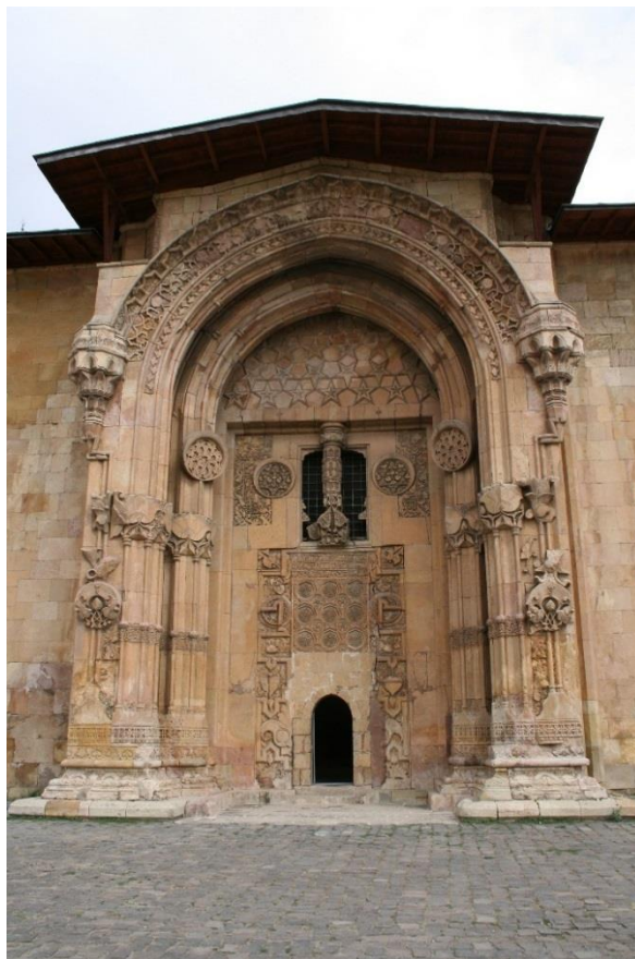
Figure 15 The main door of the hospital
