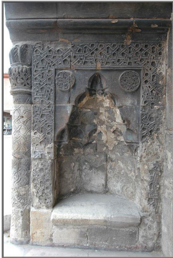
Figure 28 The main door, ornament detail
