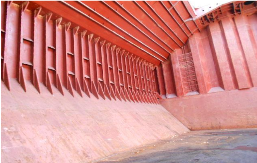
Picture 9. Hold on dry bulk vessel
