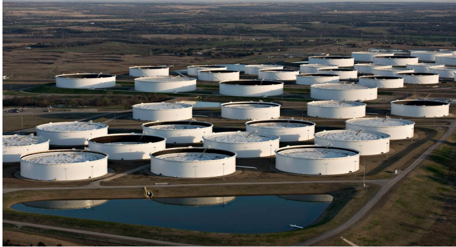
Picture 12. Tank farm
