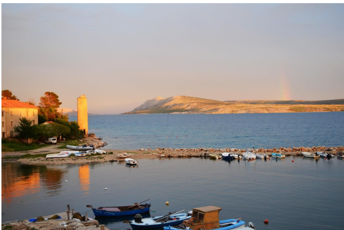
Fig. 74 Caska in the northern part of the island of Pag: the Tunera tuna watching tower and the Gulf of Pag (the salt pans of Pag are located in the background at the opposite side of the Gulf) (M. Grisonic).
