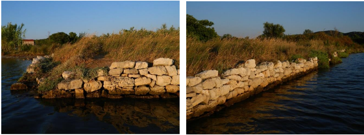
Fig. 137 Big dry wall structure on the coast – a salt warehouse?: the wall building technique (a) and the E wall (b) (M. Grisonic).
