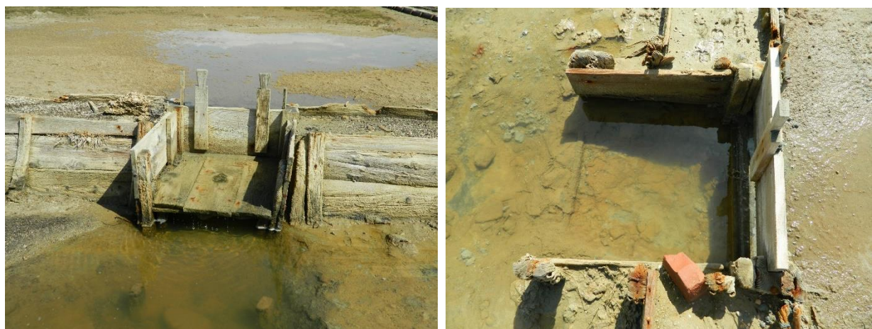
Fig. 58 Sluice gates in between the salt evaporation pools on the saltpans of Pag (M. Grisonic).
