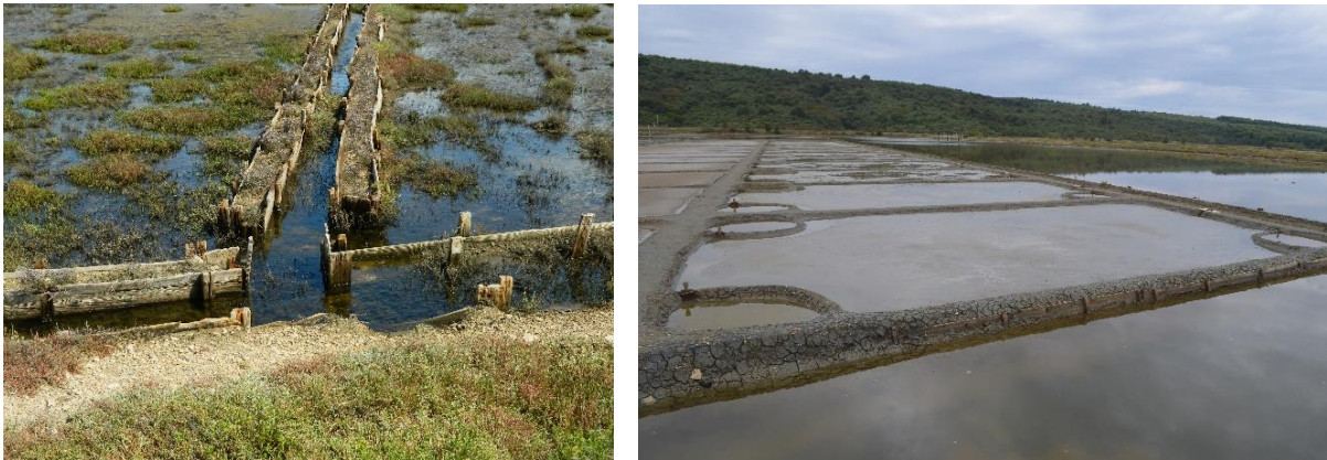
Fig. 12 Examples of embankments on saltpans: the abandoned saltworks of Dinjiška, island of Pag (a) and the still-functioning traditional saltpans in Sečovlje, Piran, Slovenia (b) (M. Grisonic).
