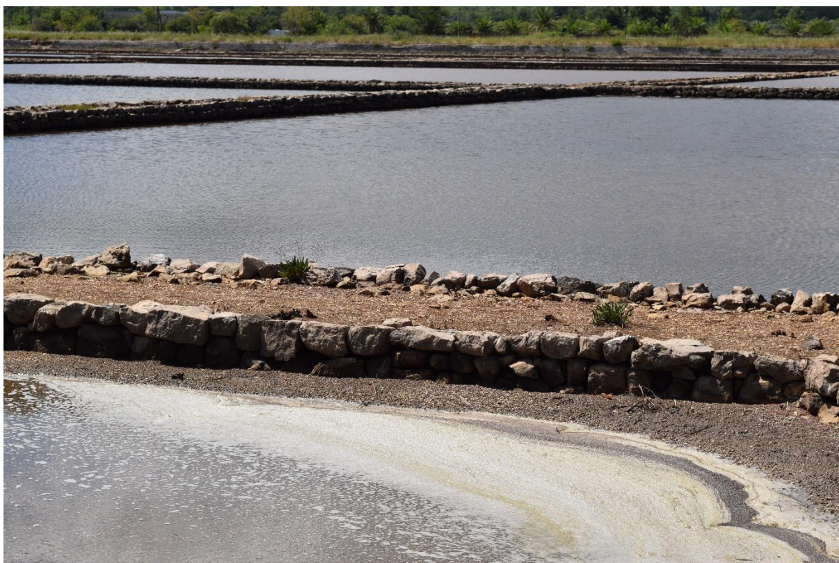
Fig. 73 Saltpans in Ston: detail of the embankments (M. Grisonic).
