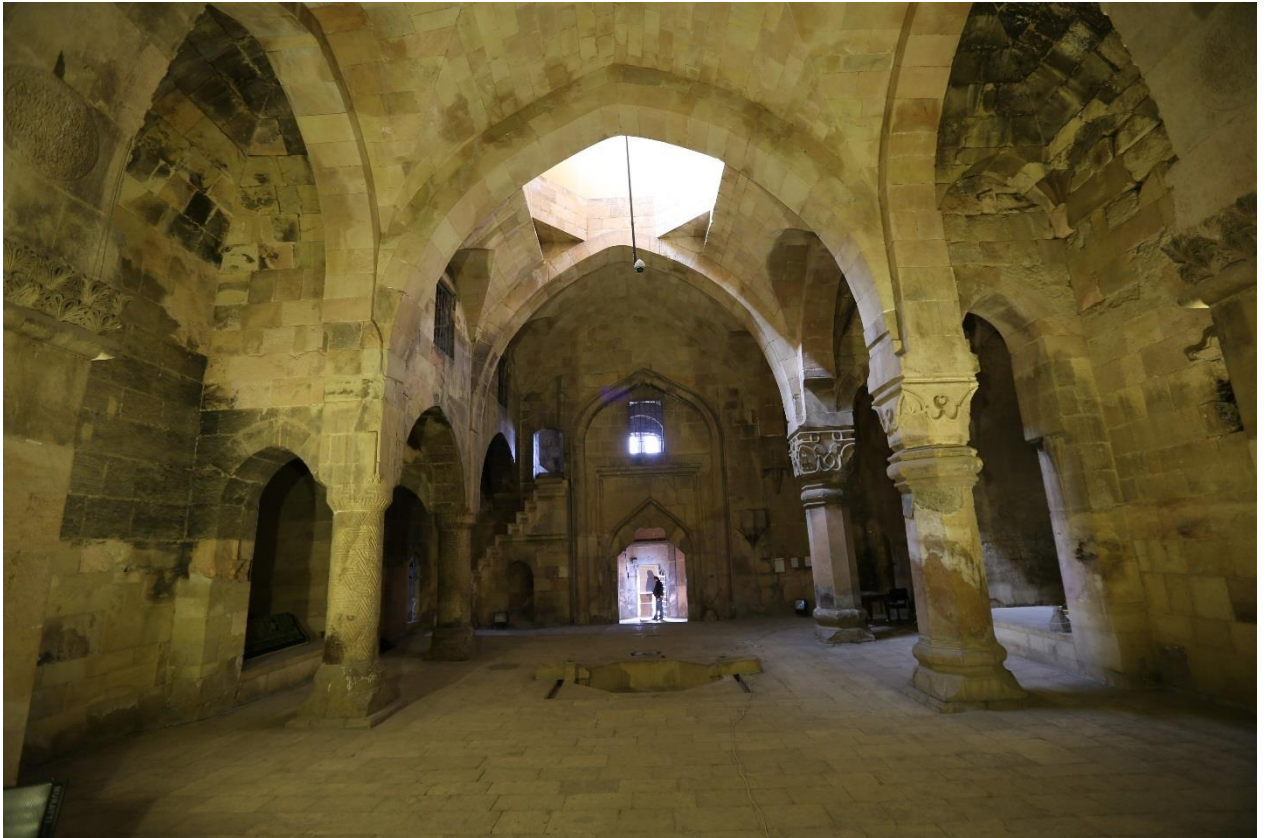
Figure 18 Inside the hospital, looking to the west
