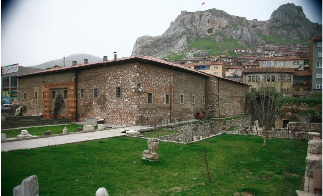
Figure 30 General view from the east
