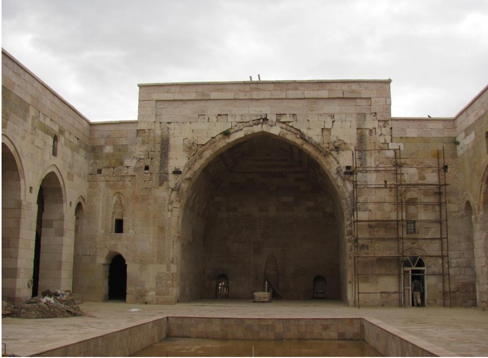
Figure 10 The main iwán and the pool, general view from the west
