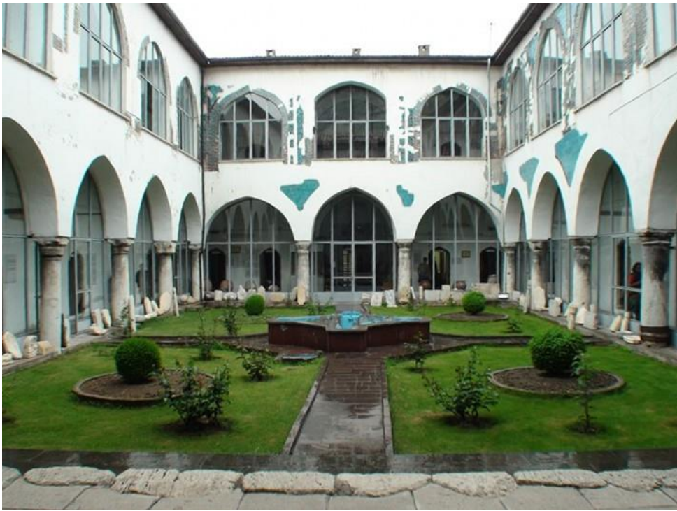
Figure 33 Open courtyard, looking at the east side
