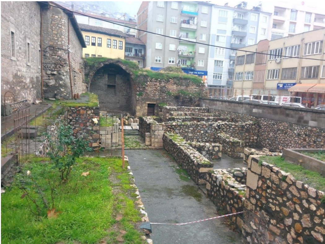
Figure 31 General view of the building from the north (Hospital?)
