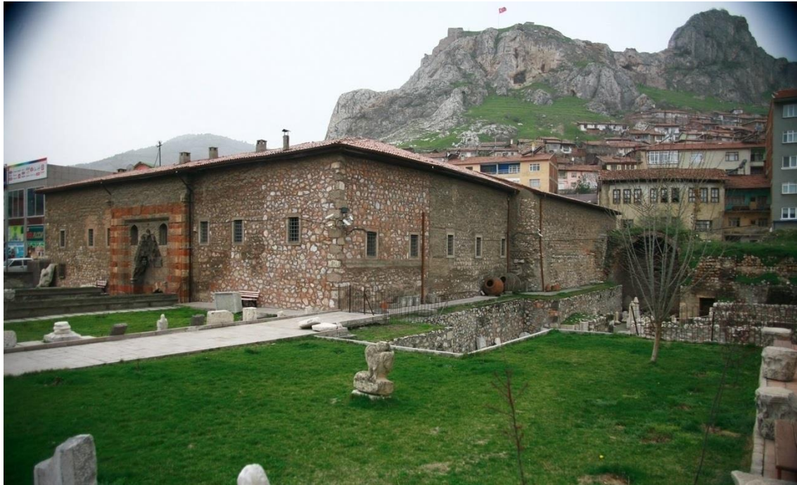
Figure 30 General view from the east
