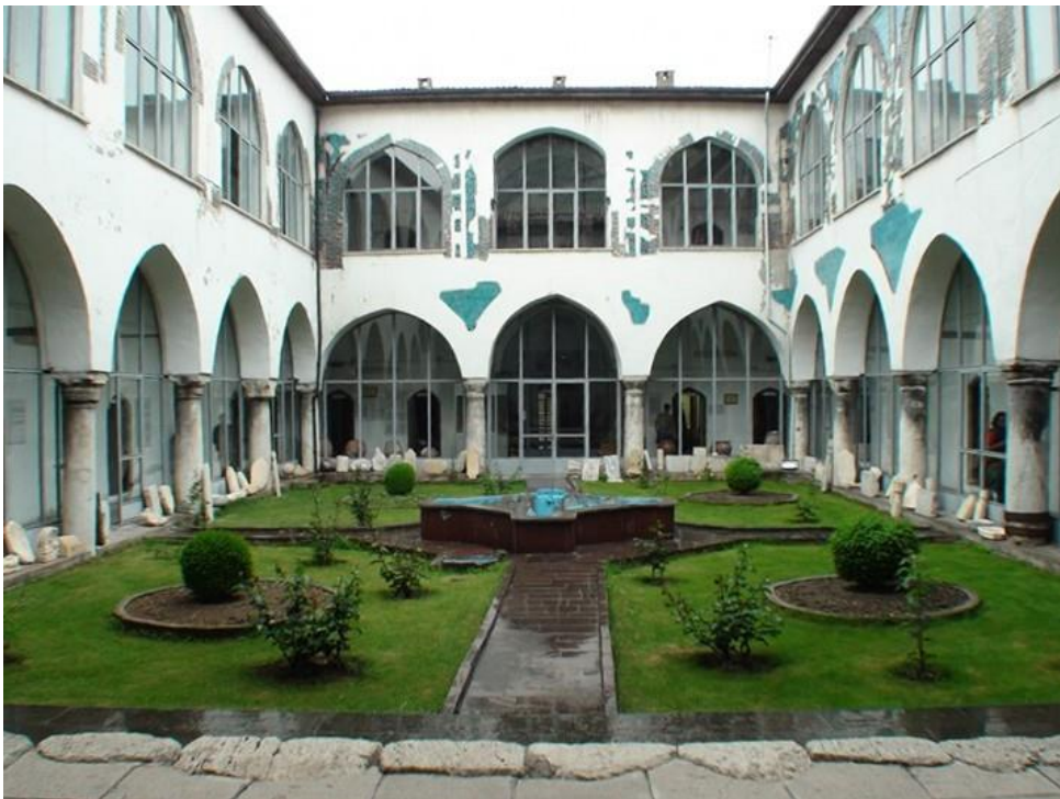
Figure 33 Open courtyard, looking at the east side
