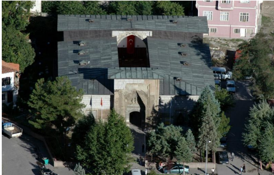
Figure 35 Amasya Hospital – General view from the west side
