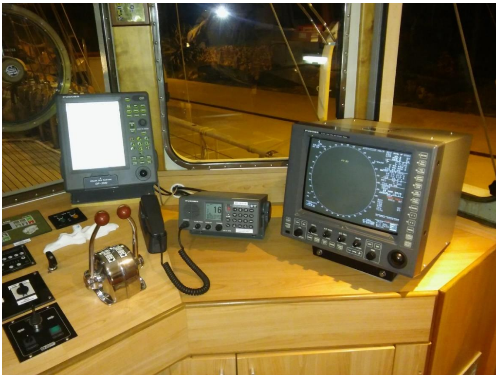
Picture 6. RADAR – Kraljica Mora
